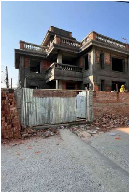
STAGE 1 Frame and brick infill complete.
