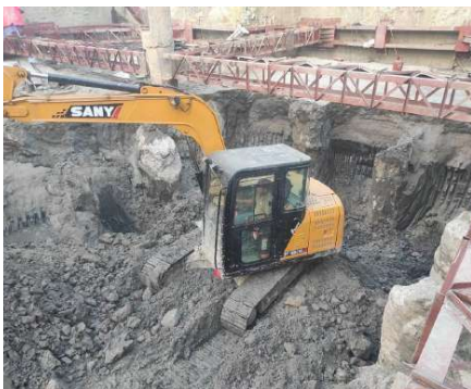
BASEMENTS Excavation behind steel strut bracing.
