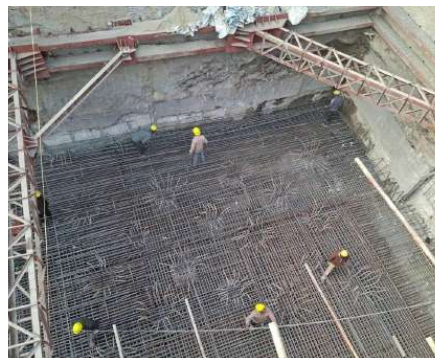
STRUCTURE Raft reinforcement before the pour.
