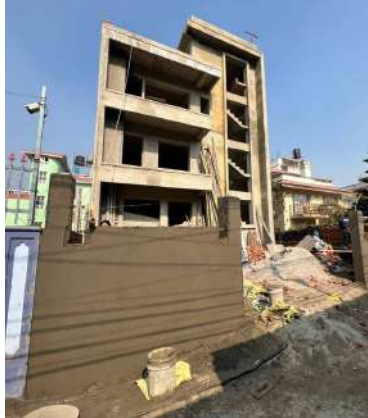
FRAME RCC frame up to the roof.
