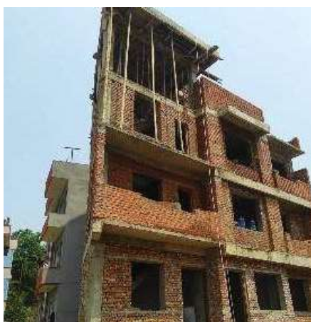
BEFORE • FRAME Brick infill on the RCC frame.
