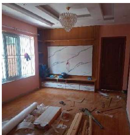
INTERIOR Living room with false ceiling.
