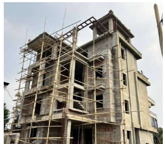
FRAME Structure complete, finishing to follow.
