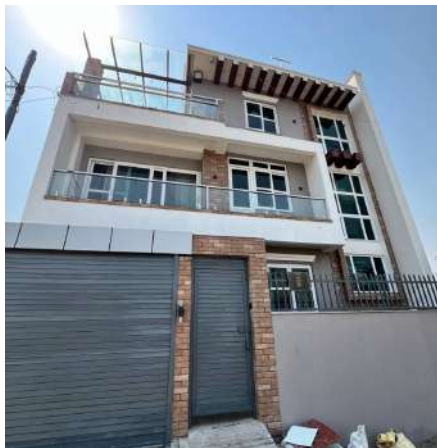
THANKOT Turnkey construction.
