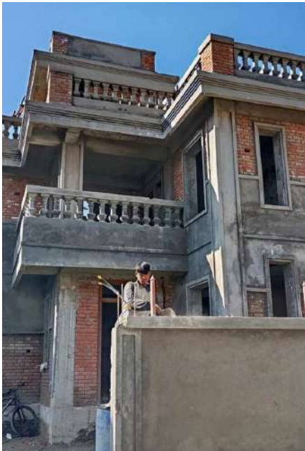
STAGE 2 Plaster and balustrades going on.
