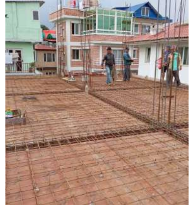
SLAB Reinforcement before the pour.
