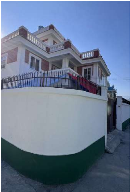
STAGE 3 Finished, with the boundary wall painted.
